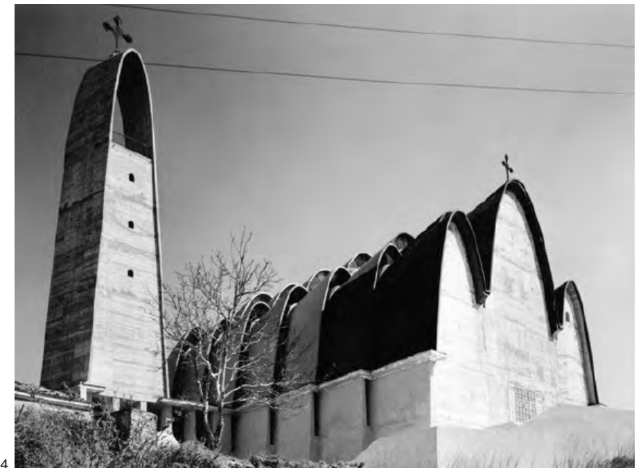
1 Interior detail 2 skylights 3 Interior view 4 Front facade and bell tower
